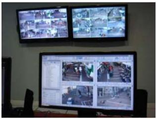
All control center operations are monitored and managed through Vigilant's Video Surveillance Suite which includes Netstream IP encoders, NetView Control Center, NetView Command, ViewStation and Remote Gateway. The system stores two weeks of recorded images in 4CIF full resolution. This technology will allow cost-effective, modular growth by updating the components according to the needs dynamically.
